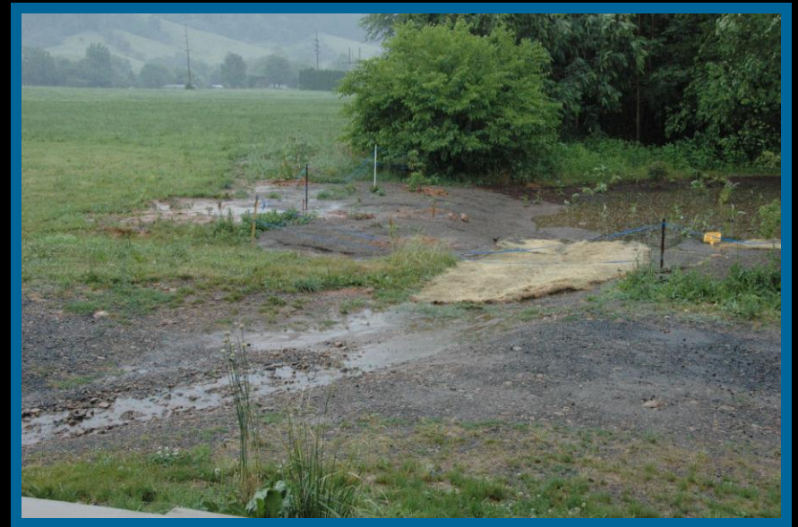
RappFLOW's Rain Garden, showing the path of run-off flow
